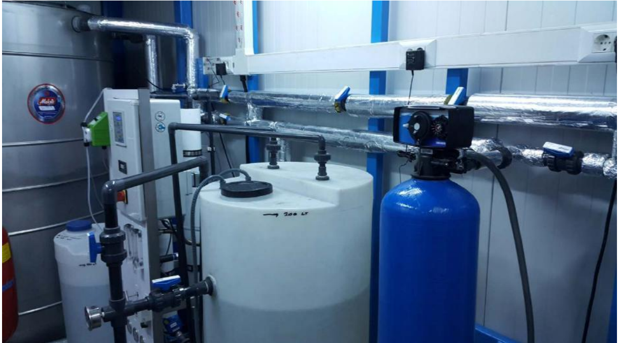
TEKFEN CONSTRUCTION — TANAPPROJECT COMPRESSOR and MEASUREMENT STATION (CS1)CAMP — POSOF-ARDAHAN/TURKEY — Potable Water Treatment Plant, 112.5 m 3 /Day (2016)
